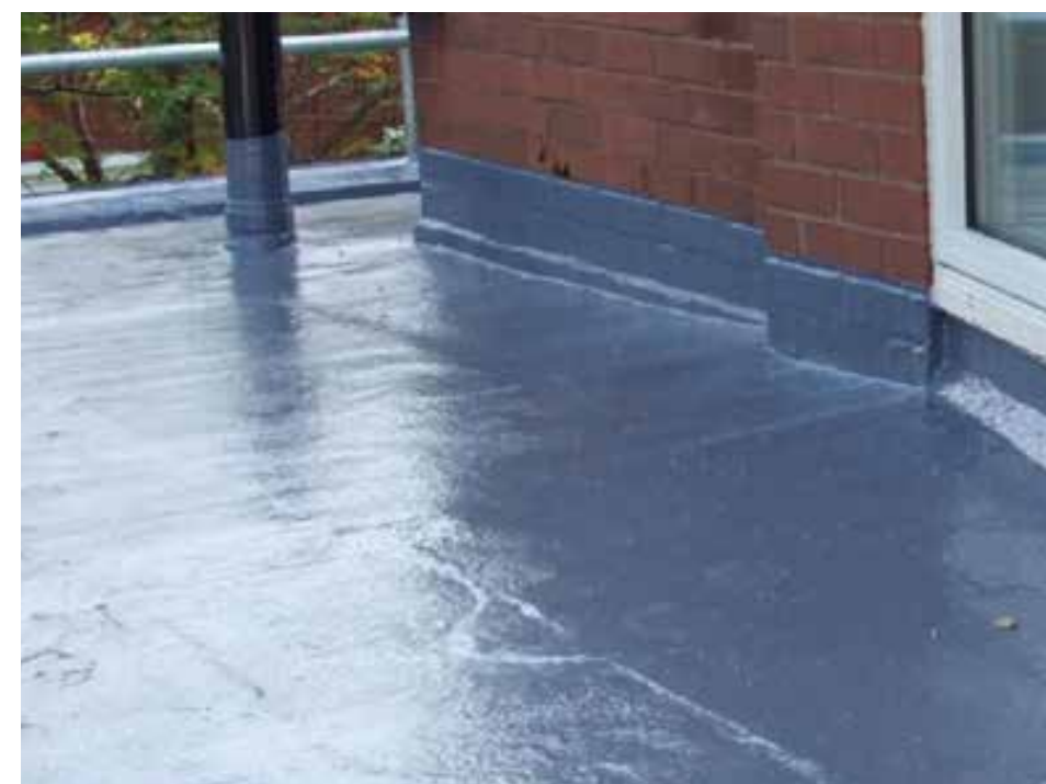
Liquid applied waterproofing
