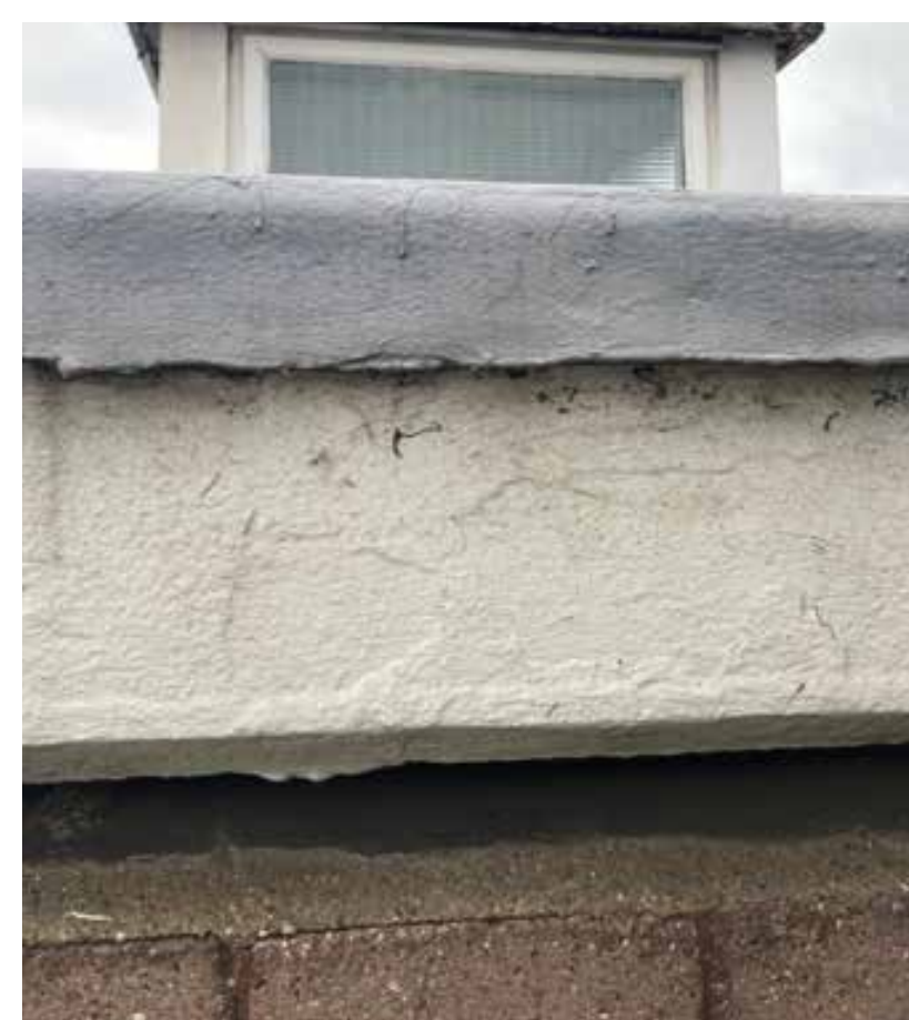
Asphalt waterproofing visible on front of roof slab
