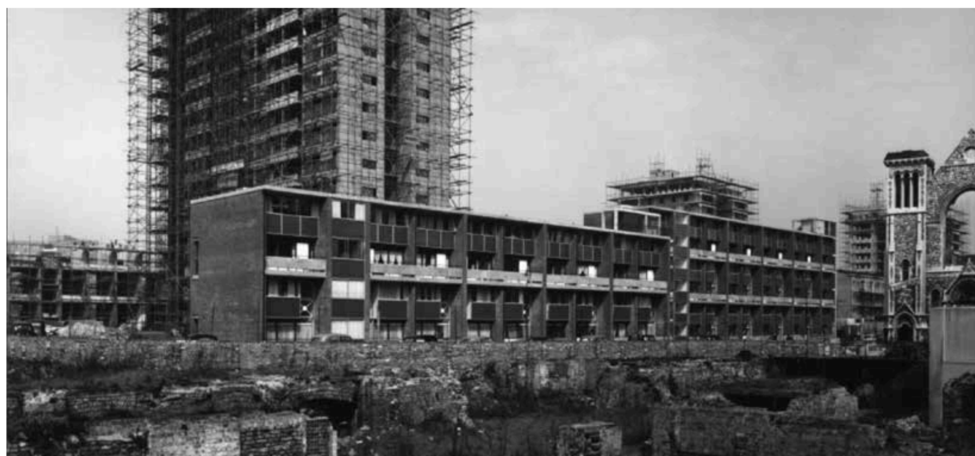
Archive photograph showing the recently completed building with crisp concrete edge profile
