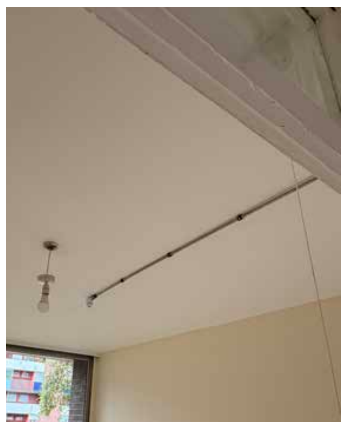
4. Exposed pipework to be painted white
