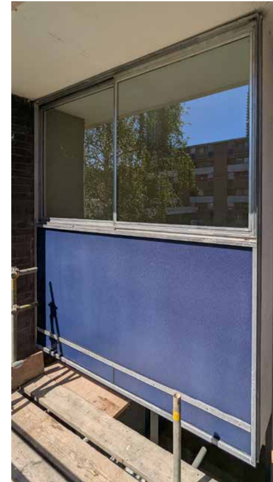
Above: Trial works to horizontal sliding window in bedroom. The frame inserts, vacuum glass, stainless steel bearing (not visible) and new blue glass have all been installed.
