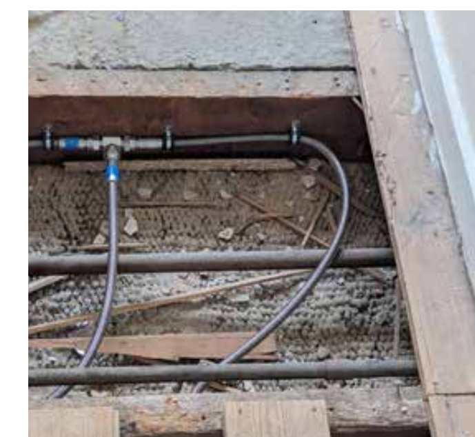
3. Pipework run in floor void
