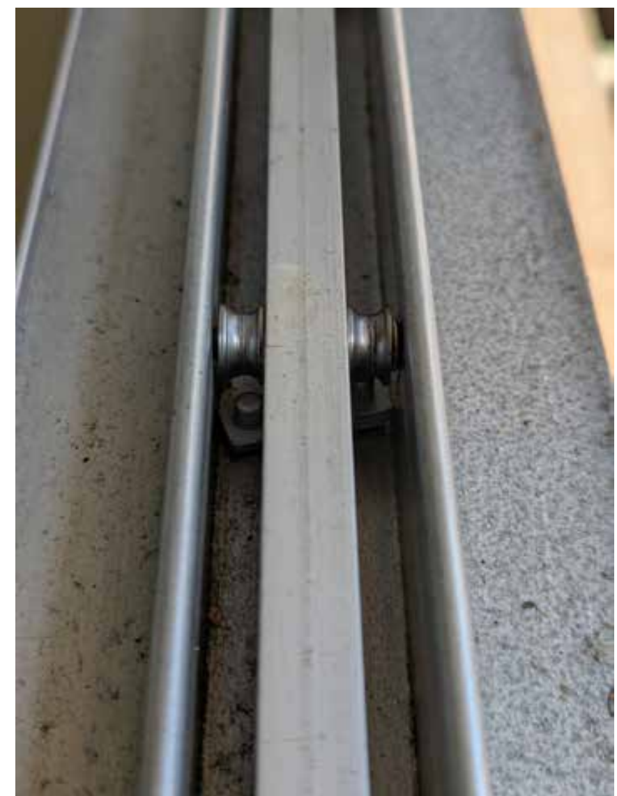
Right: Trial works to bedroom horizontal sliding window showing new stainless steel bearings installed to bottom of window frame.
