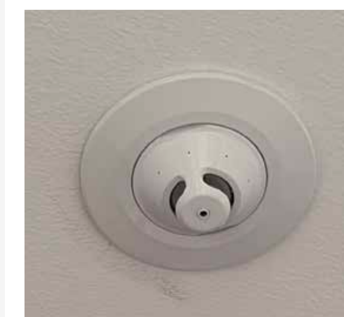
1. Recessed mist suppression heads (m1 on drawing)
