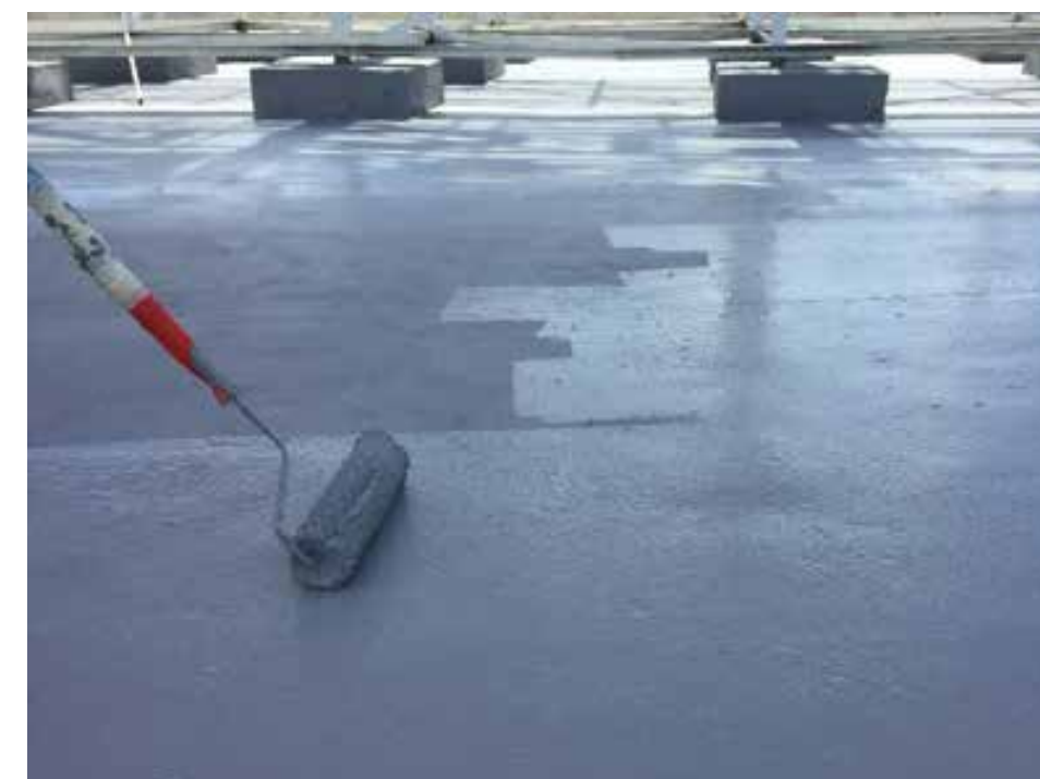
Application of waterproofing
