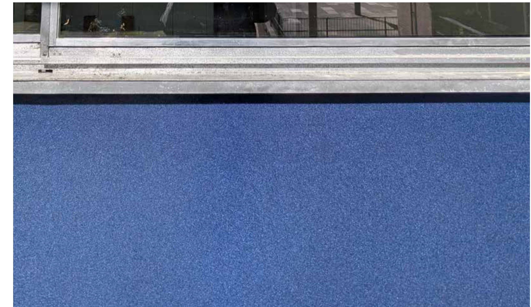
Replaced spandrel panel installed for the 2 Bayer House trial. The replacement glass is a bespoke design with a textured outer face and a blue ceramic coating to the rear.
