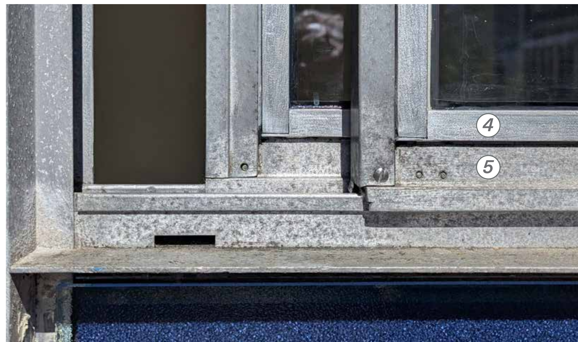
Left: New aluminium glazing adaptors installed for trial.
