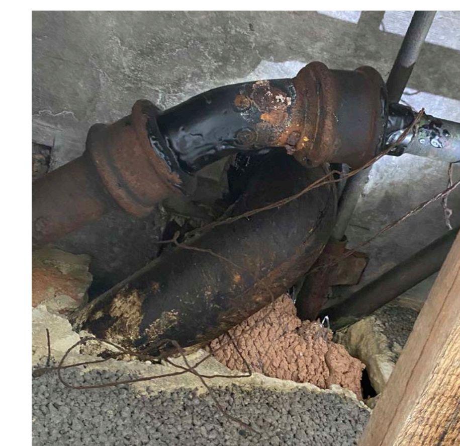
Metal wire mesh and bonding plaster with significant gaps.
