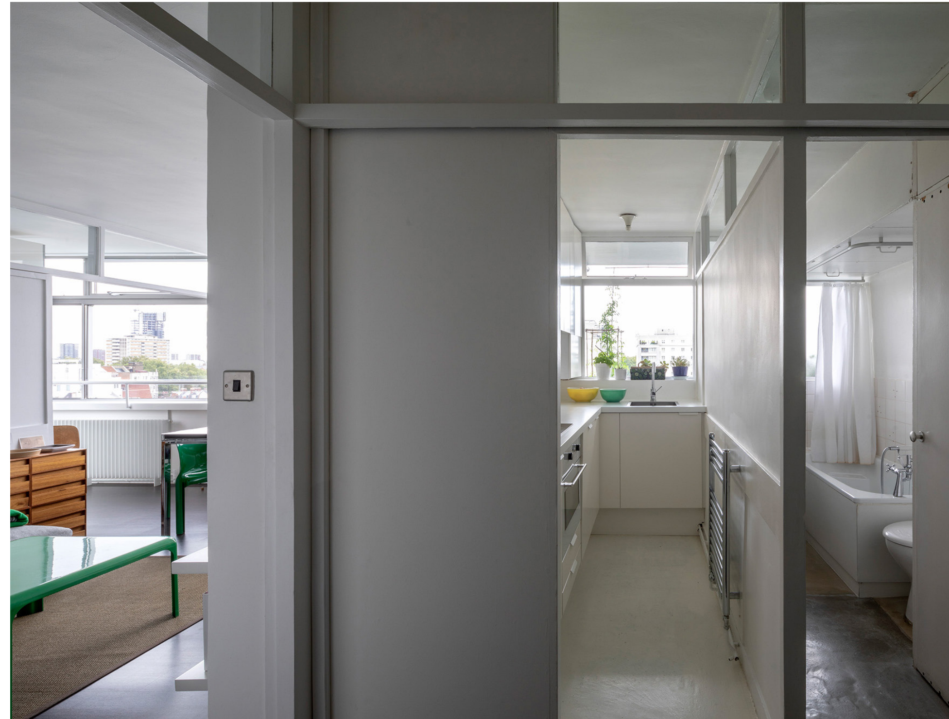
Full height timber glazed partitions separating the living room and bedroom, including the original sliding partition, and the fixed glazed partition between the kitchen and bathroom.
