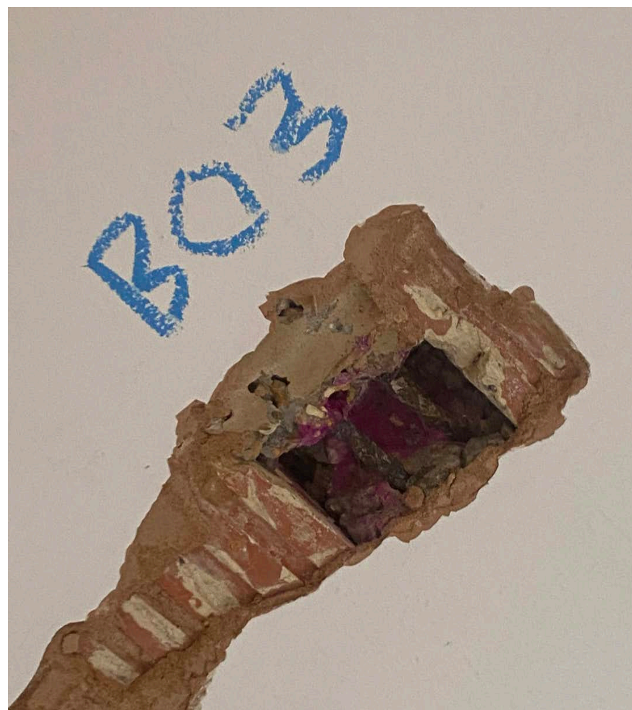
Steel in the reinforced concrete ribs with poorly compacted concrete carbonation.
