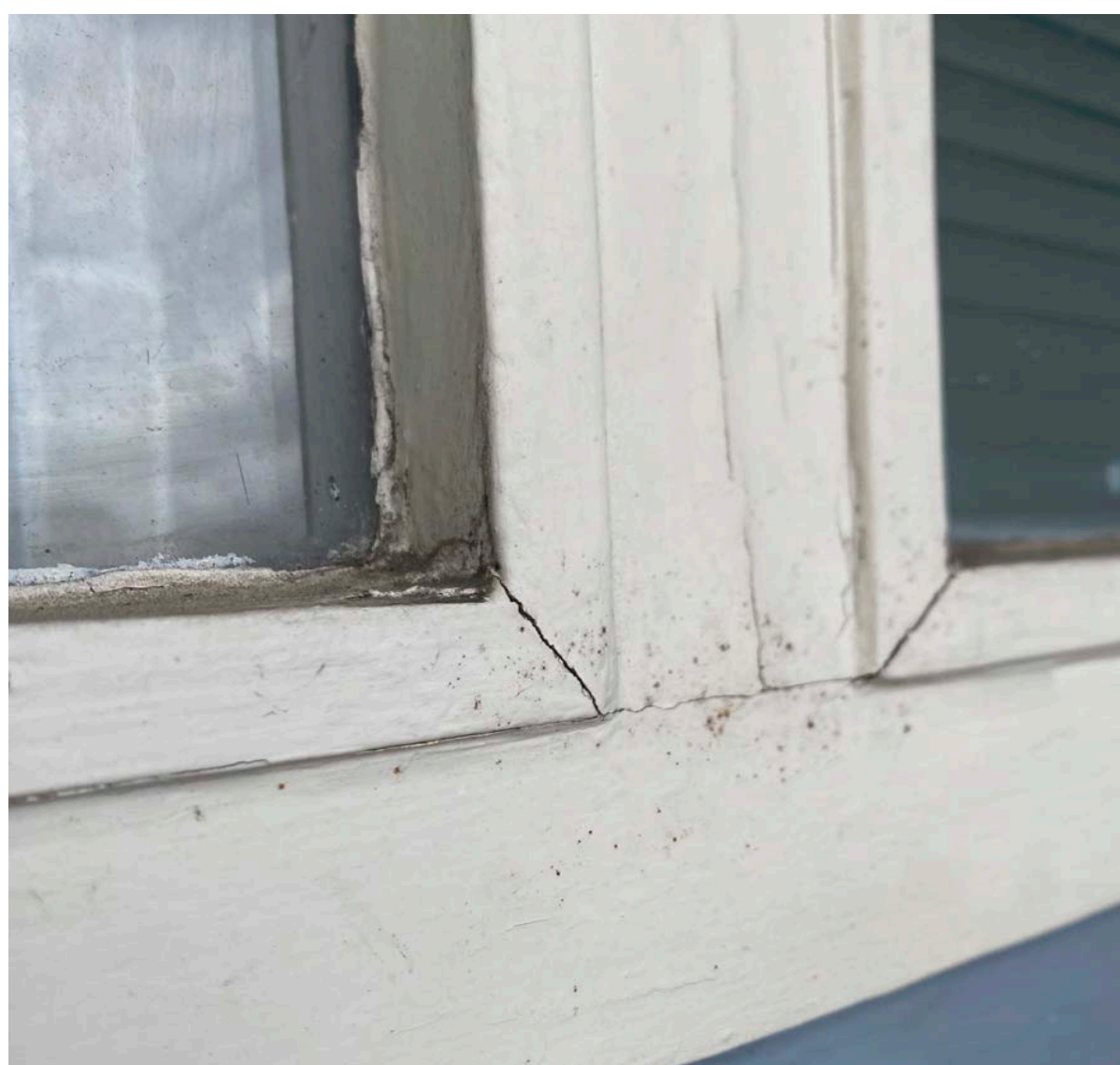
Timber beading projects out from the frame.
