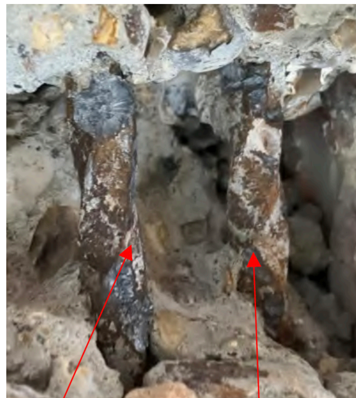
Steel in the reinforced concrete ribs with poorly compacted concrete carbonation.
